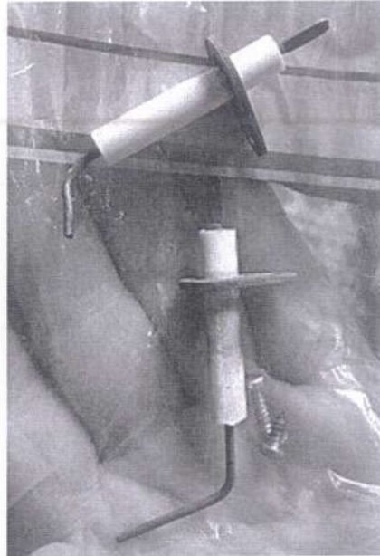
Figure 8: Flame-igniter (top)-and-flame-sensor
